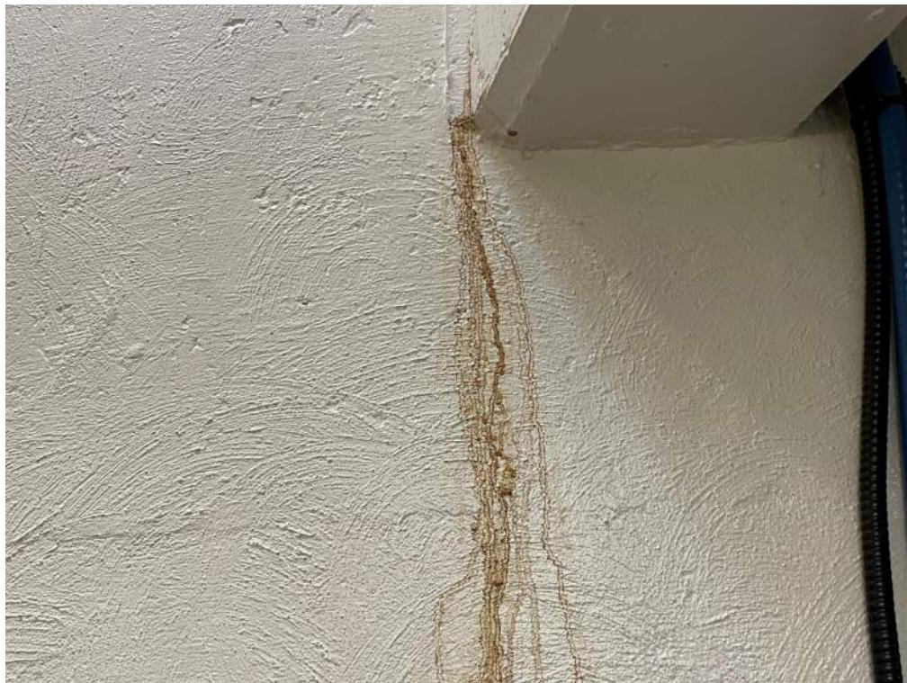
Photo 11: Leaking from roof in original control building
