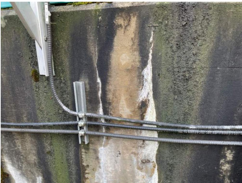
Photo 19: Efflorescence at north RBC wall
