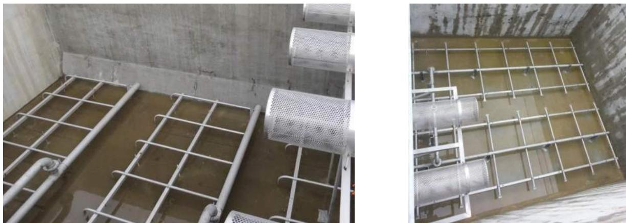
Figure 3      Aeration grids & MBBR Sieves
