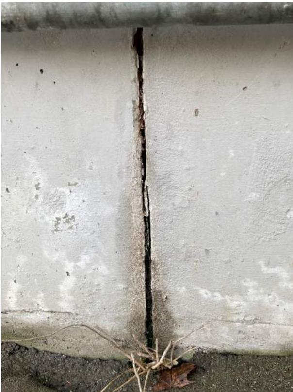
Photo 17: Cracking at west construction joint between grit tank and sedimentation tank 1
