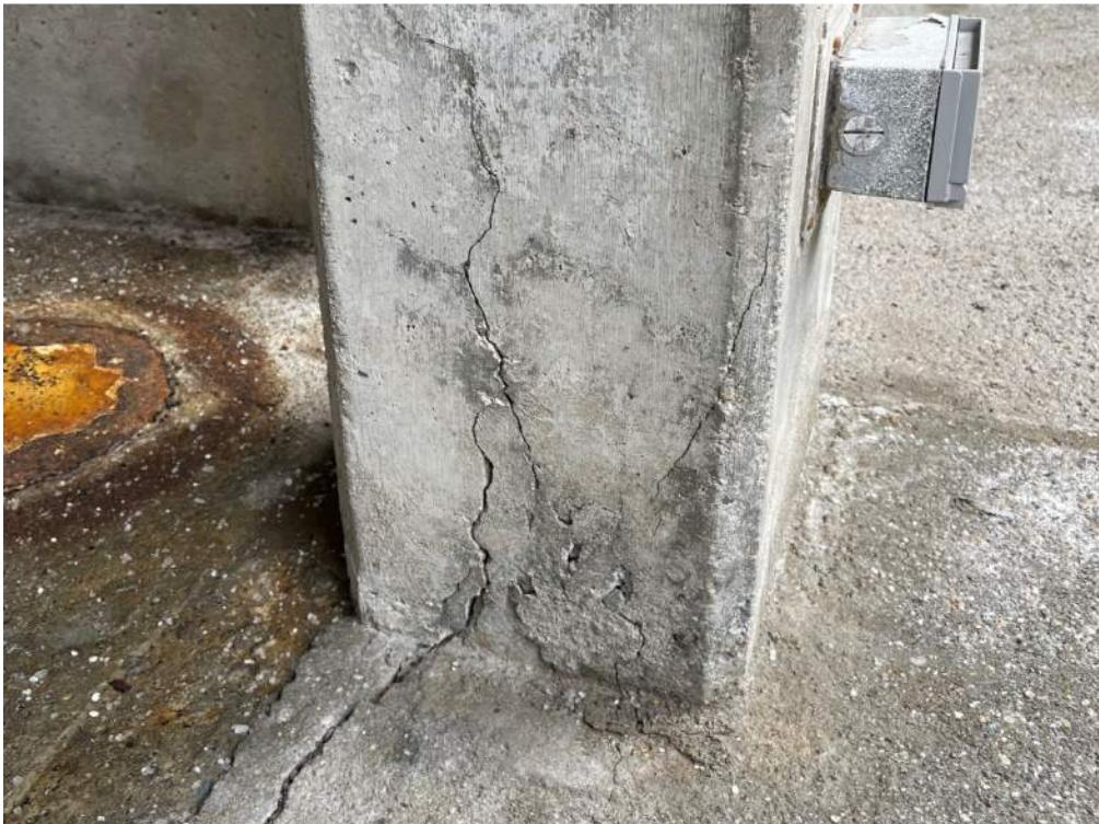
Photo 16: Cracking at column between grit tank and sedimentation tank 1
