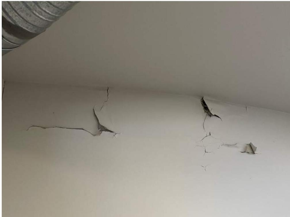
Photo 12: Leaking from roof in original control building
