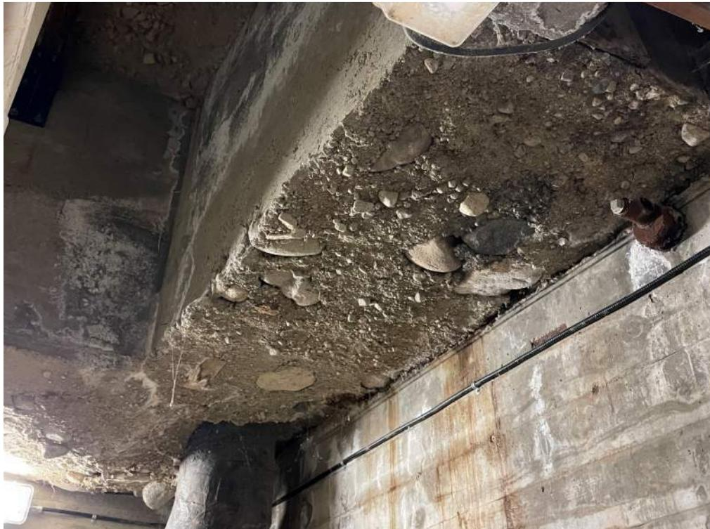
Photo 14: Excavation under existing foundation
